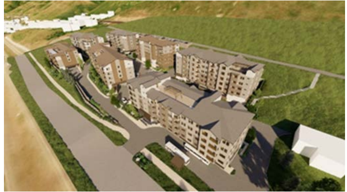
West Timber Ridge
