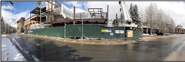
Progress on Vail Health East Wing Expansion
