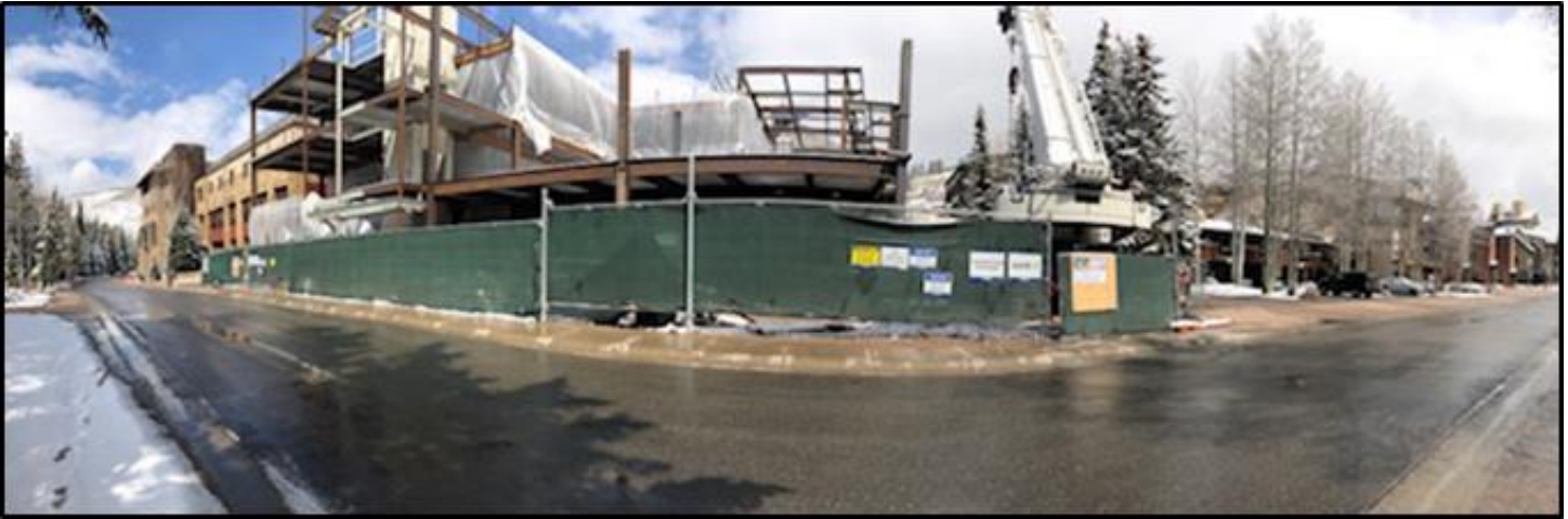
Progress on Vail Health East Wing Expansion.
