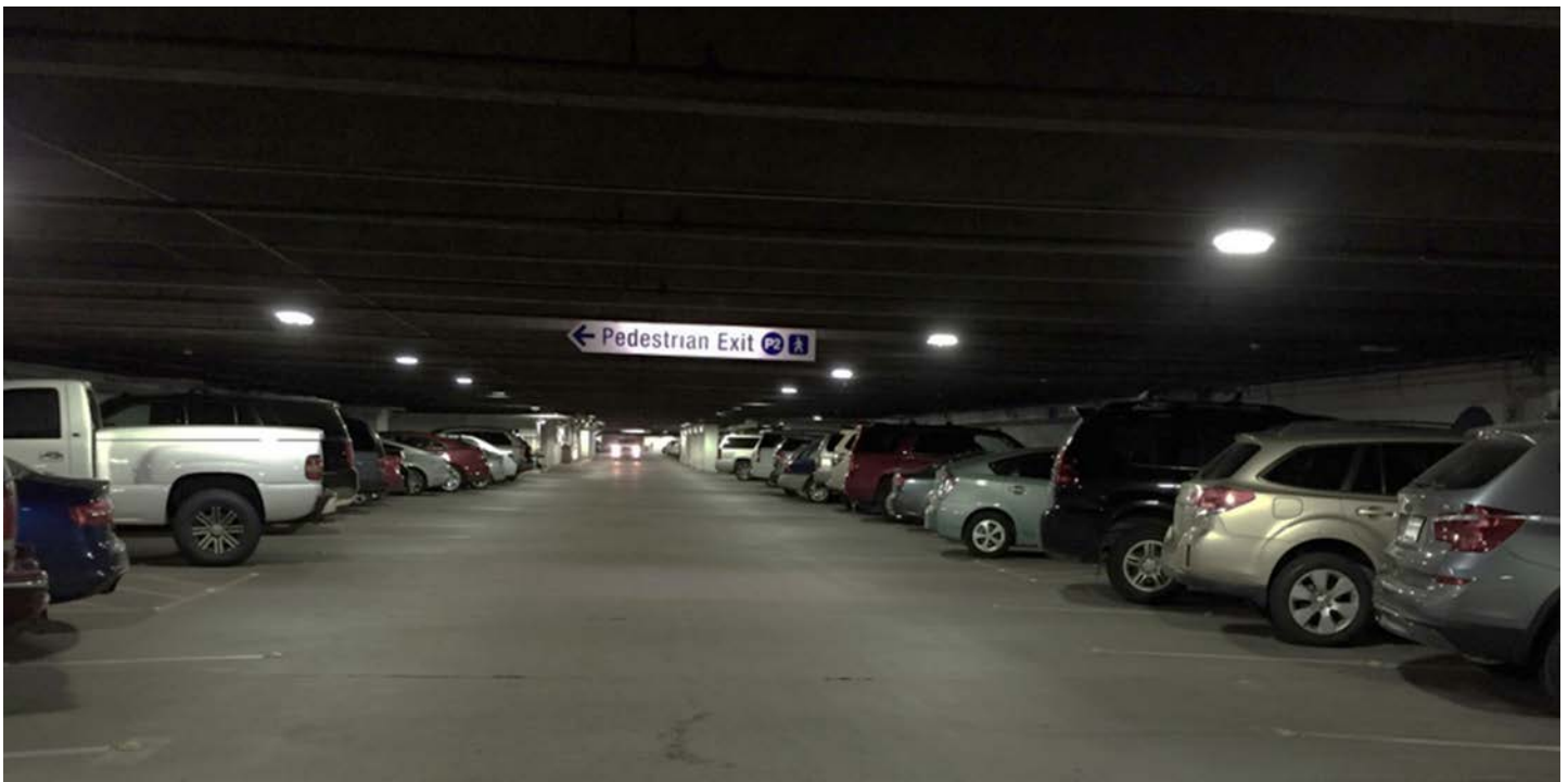
Vail's ageing parking structures are in need of being expanded and refurbished.
