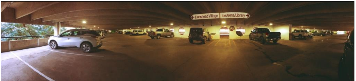
Lionshead Parking Structure – How long will it last, how much to replace?
