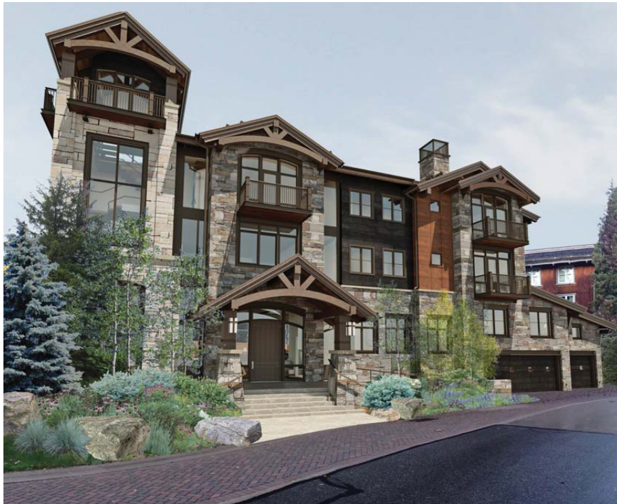
Proposed Avanti Lodge – 366 Hanson Ranch Road – Developer: VailPoint LLC. Contesting Open Space Covenant Protections
