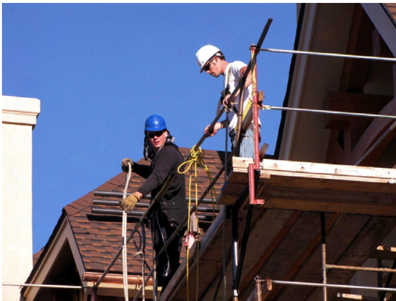
Lions Square Lodge North construction
