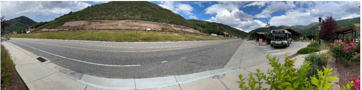
West Middle Creek Subsidized Housing under construction.
